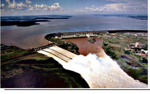
World's largest hydroelectric plant (until China's 3-Gorges), converts potential energy of water to K.E., and then electrical energy(Ch.25); Recall, form of solar energy (why?)
